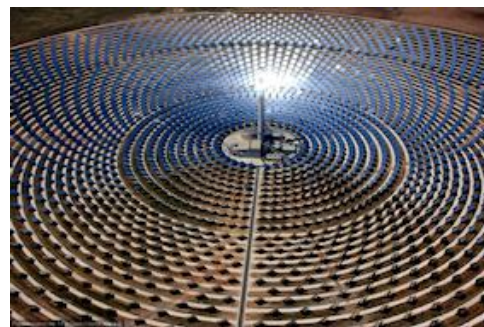
Crescent Dunes (Nevada, USA), 2015
