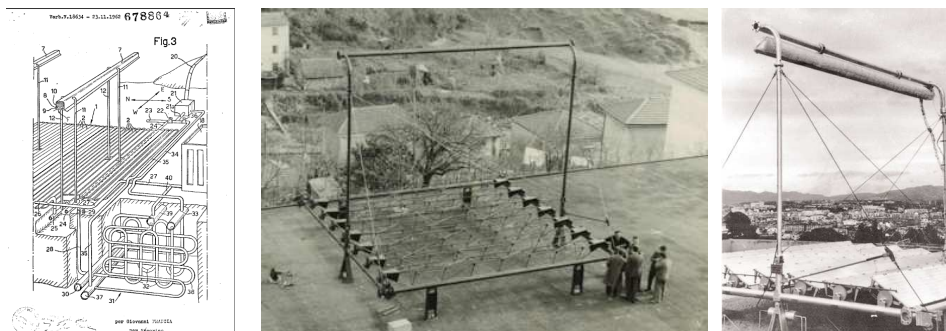
Fig. 6. Left: drawing of the patented LFC; Right: Photos of Francia's first LFC prototype (Francia Archive, Musil Brescia).
