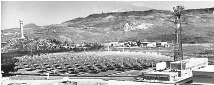
Fig. 1a, b: Two views of the 1 MW Eurelios power plant at Adrano, Sicily. The central boiler rises above a field of mirrors. This was the world's first example of solar kWhs being fed into a national electricity grid. The project was undertaken jointly by ENEL and the European Economic Community (Photo ENEL).
